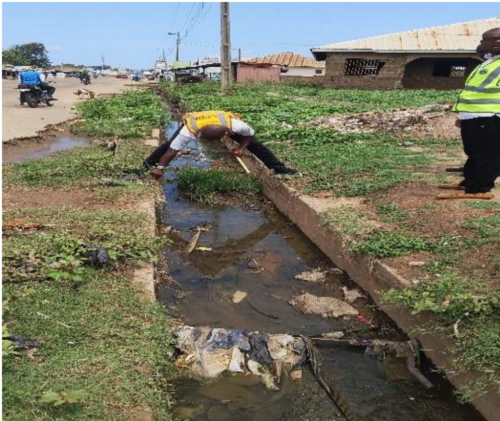
Figure 1. Field assessment of a roadside drainage channel..
